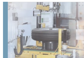
Retrofit of balancing line RTB Page 41
